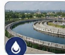
WATER & WASTEWATER TREATMENT PLANTS
