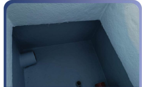
MANHOLE LINING Chemical & water resistant protection
