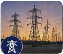
POWER PLANTS & SUBSTATIONS
